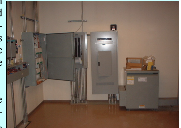
End Results—early meticulous planning bore fruits after concrete was poured.
